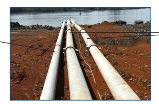
Sphere Lock couplings allow for angled/offset connections.
