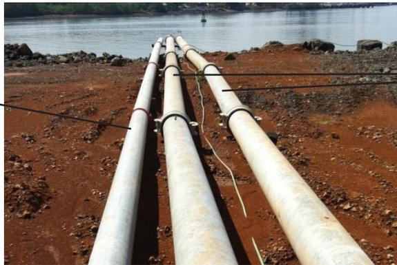
*Sphere Lock™ couplings allow for angled/offset connections.*
